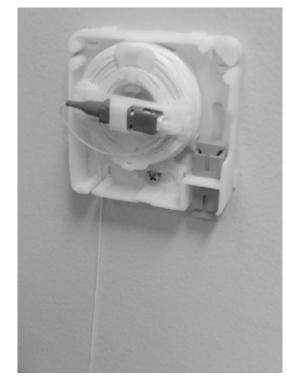
6. UNSPOOL THE REQUIRED LENGTH OF FIBER PULLING IT THROUGH THE APPROPRIATE OPENING IN THE BASE.
