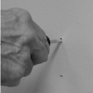
2. USE THE PHILLIPS #1 SCREWDRIVER TO PUNCH TWO HOLES IN THE WALL OR DRILL WITH 5MM OD DRILL BIT AT THE TWO MARKS.
